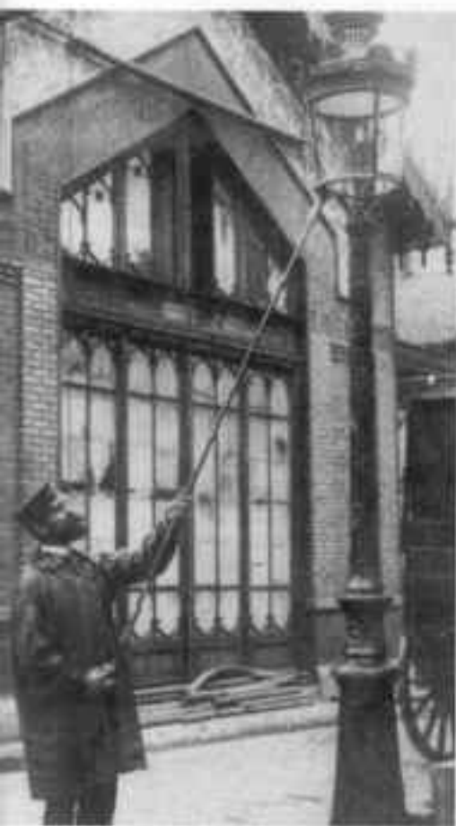
Gas street lamps.
